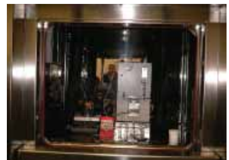
Figure 17: Hot cell. (Source: CHUS Facility)
